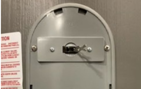
The lower element disconnect in the OFF position. (To the right)
